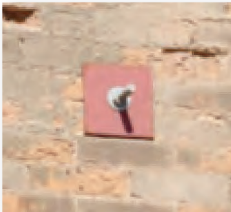
A steel plate with anchor bolts.
