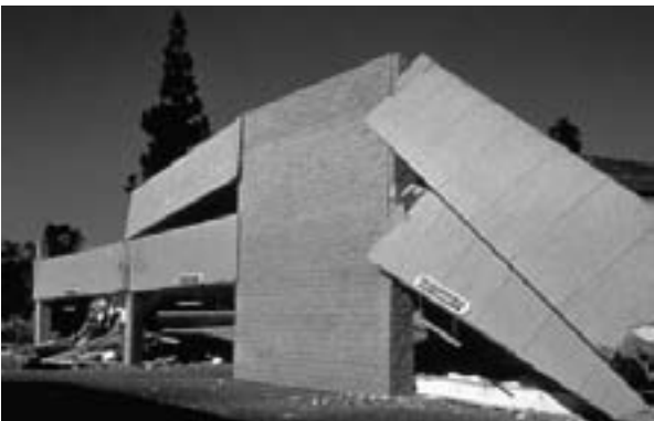
Figure 5 - Concrete Parking Structure Collapse.
