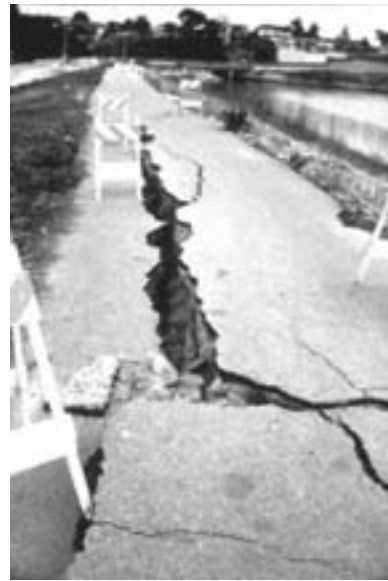
Figure 67 - Lateral Spreading. Loma Prieta Earthquake, October 17, 1989. Lateral spreading damage levee road along the San Lorenzo River.
