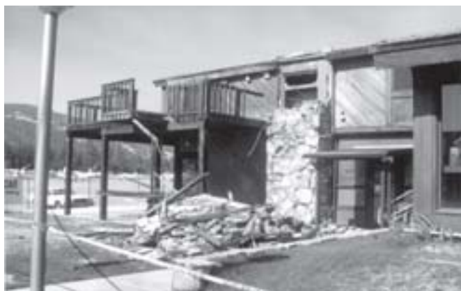
Figure 35 - The chimney on this building fell on the stair-way in the 1992 Big Bear earthquake, cutting off a means of escape for persons on the second floor.
