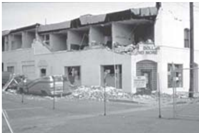
Figure 16 - The second-story wall of this unreinforced masonry building was not well-tied to the roof, and the building collapsed during the 1994 Northridge earthquake.
