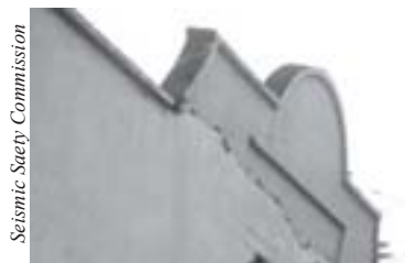
Figure 18 - Parapets. They are the tops of walls above the roof can fall off buildings like this one nearly did in Rio Dell during the 1992 Cape Mendocino Earthquake.
