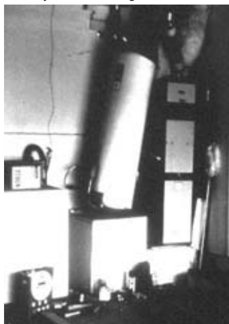
Figure 11 - This unstrapped water heater tipped over during the 1984 Morgan Hill Earthquake. Fortunately gas and water lines were not ruptured.
