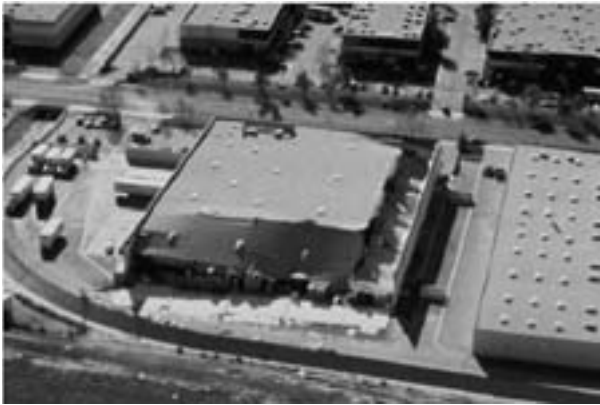
Figure 1 - Partial Collapse of an Industrial Building. Poor connections between the walls and the roof caused this collapse.
