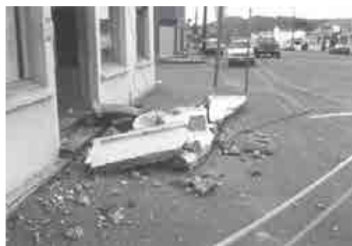
Figure 20 - Unbraced Parapets can Injure and Kill - This parapet on the front of the building in Figure 18 fell on the sidewalk.
